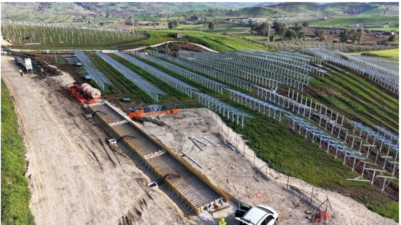
Once fully operational, the Ciminna agricultural photovoltaic park near Palermo will generate over 120 GWh of electricity annually.
