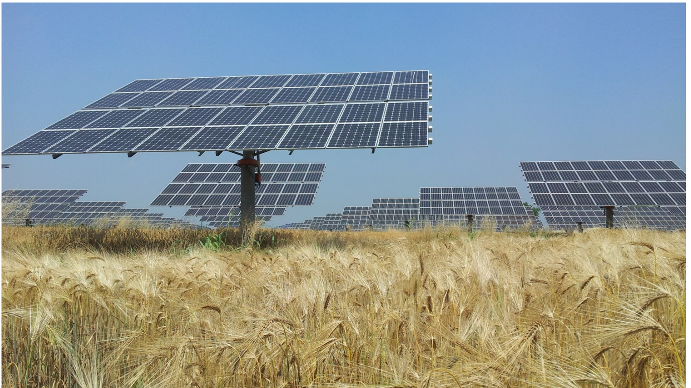
Bifacial agrovoltaic plant at Castelgugliermo.
