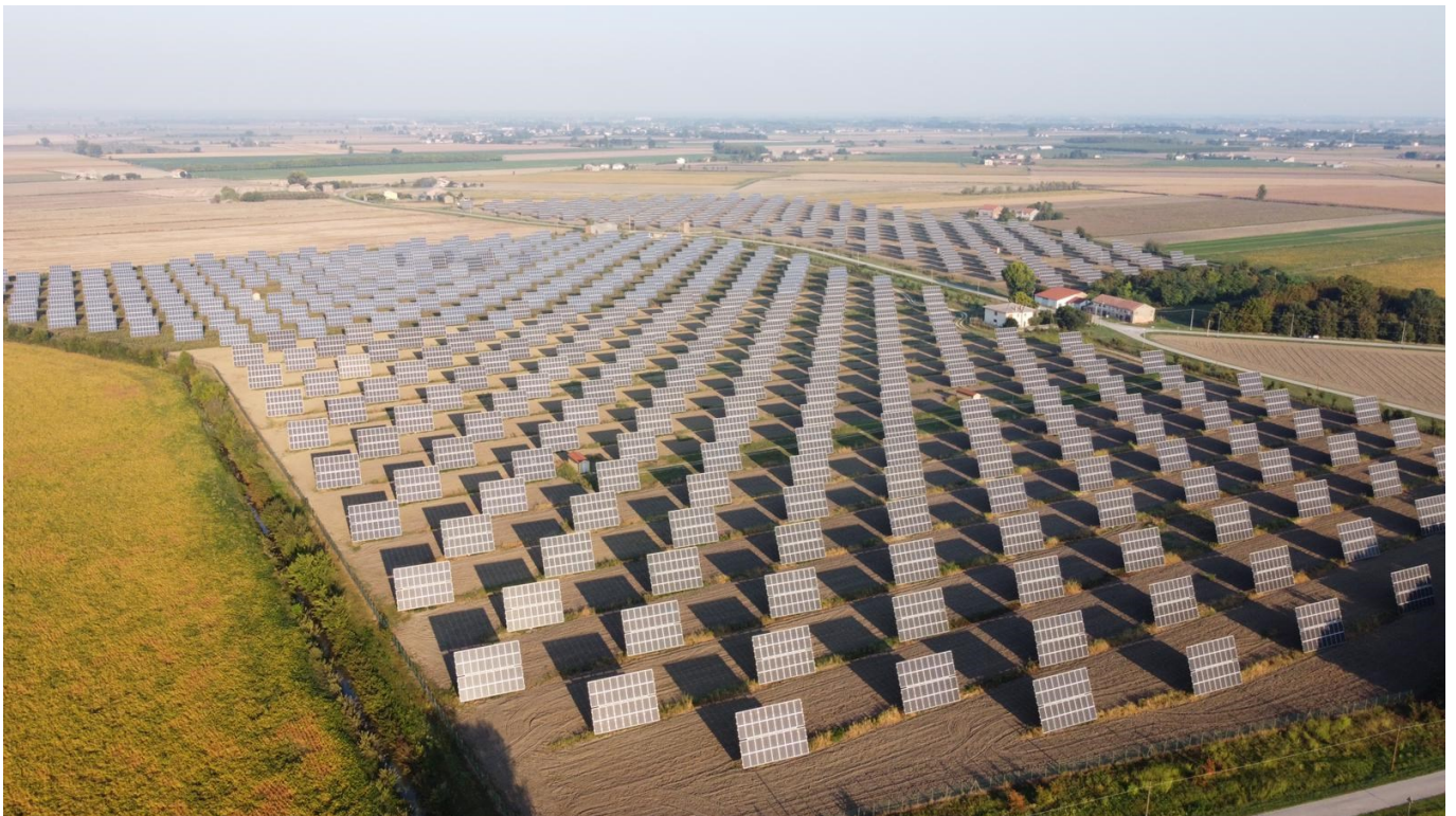
The solar power installation in Castelguglielmo has been fitted with more efficient bifacial modules.
