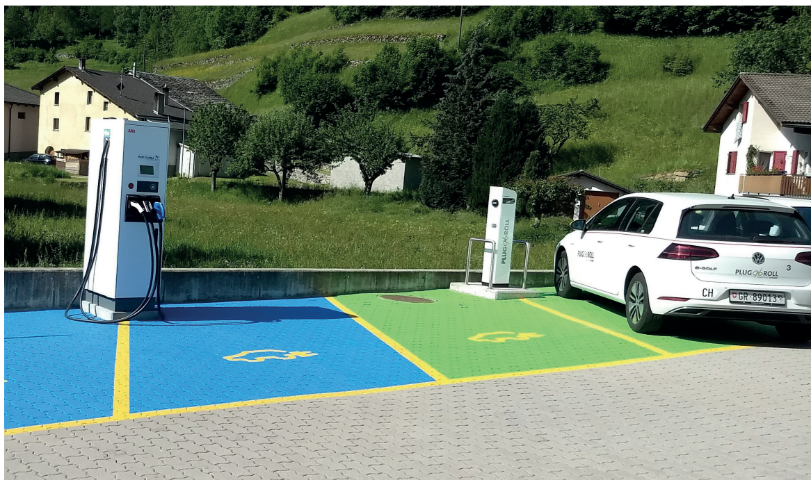
Valposchiavo's first rapid charging station
