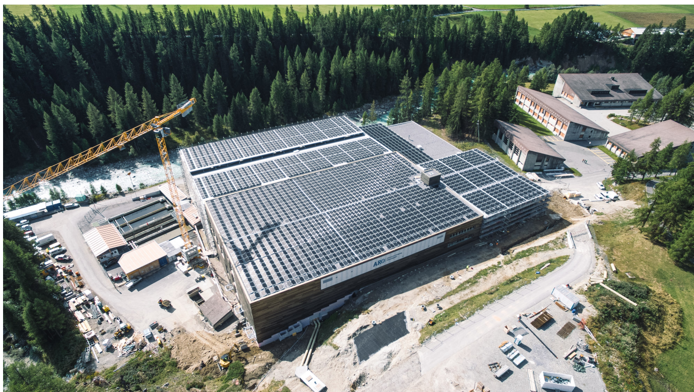
Photovoltaic installation on the roof of ARO Oberengadin sewage treatment plant
