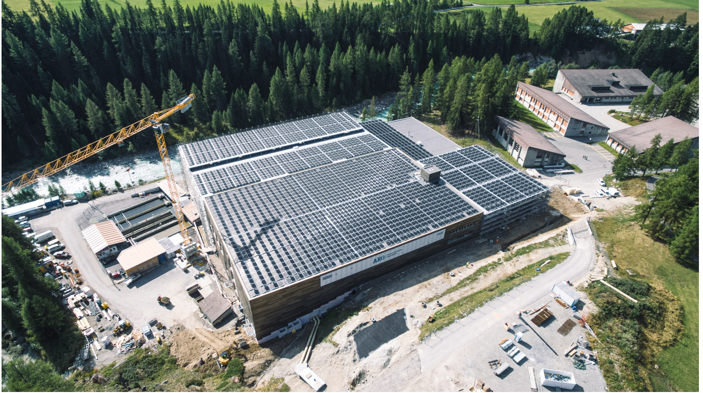
Photovoltaic installation on the roof of ARO Oberengadin sewage treatment plant
