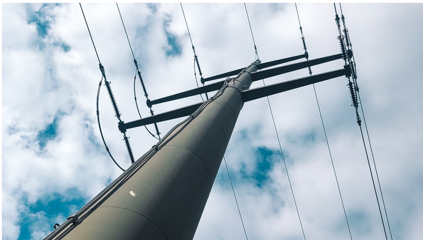
High-voltage twin cable line in the Surselva
